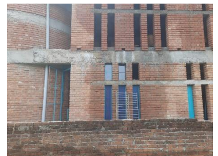
Our windows will be in shades of blue and green. They open on a central pivot like a shutter. The upper windows in each floor will be clear fiber sheets.
