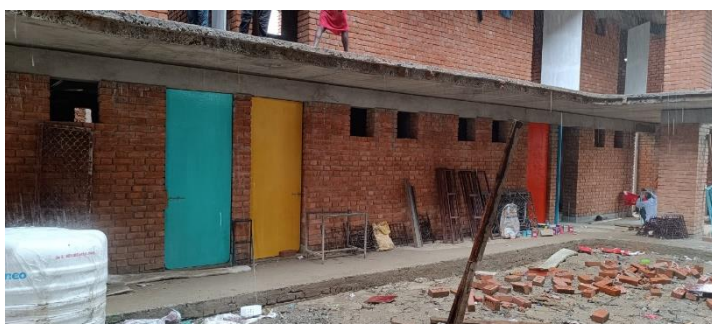
The first doors painted
