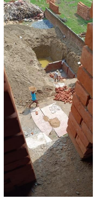
Septic tank in progress
